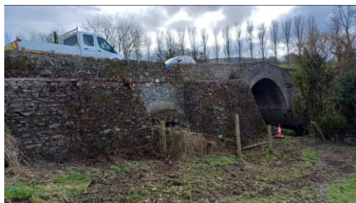
George's Bridge, Ballintruer More
