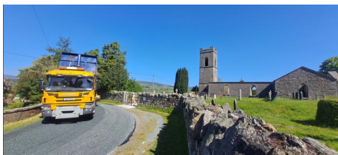
Surface dressing at Derrylossary, Roundwood.
