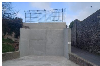
Handball Alley refurbishment
